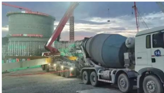
Concrete is poured into the conventional island's inner retaining wall (Image: CNNC)
